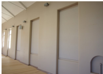
Reduce Noise in Multi Purpose Halls
