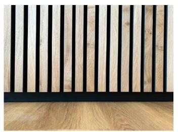
Decrasound Decraslats are an Acoustic Wall Panel System consisting of a combination of DECRATIMBER decorative timber wall linings and ACOUSTISCREEN polyester fibre sound absorbing panels.
